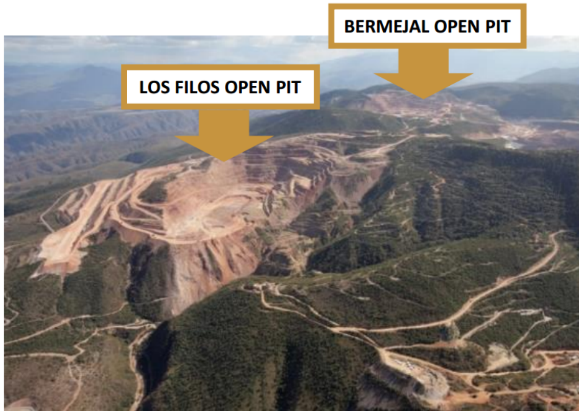
Aerial view of operations
